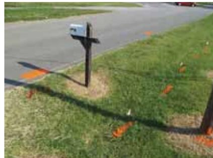
*Offset marks on street provide actual location information based on measurements in case locate marks are wiped out.*
