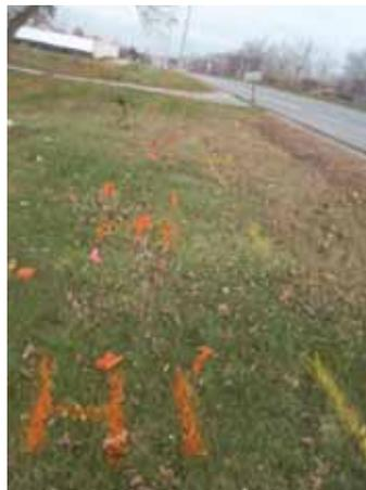
*Proper gas main markings with improper conduit marks for electric and communications*
