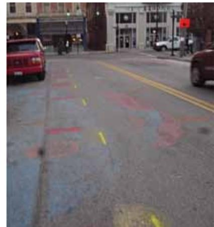
*Communications conduit to the left, direct buried phone (center) and on the right, a gas distribution main.*
