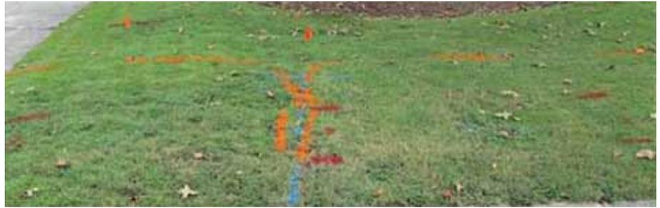
*Marks, without proper flags, showing 4 lines marked using proper color codes for telecommunications (orange), power (red) and water (blue).*
